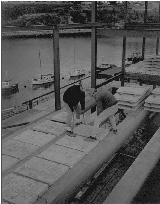
Figure 4.6: Composite beam and plank floor under construction.
