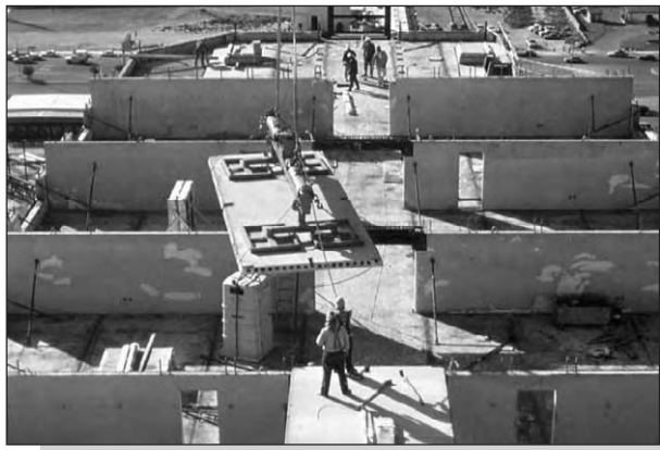
Figure 3.3: Wall frame with 3.6 m wide hollow core floors (courtesy A. Curd and Partners, USA).
