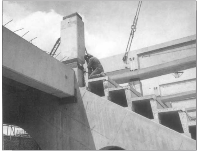
Figure 3.13: Example of H-frame used in stadia (courtesy Tarmac Precast, UK).
