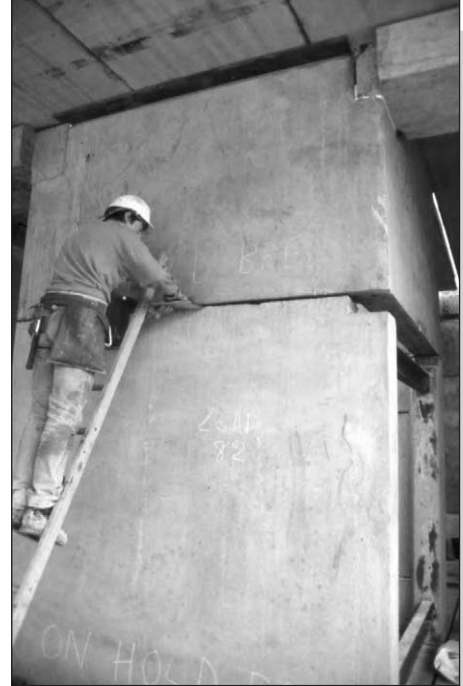
Figure 6.31: Dry packing between precast concrete walls.
