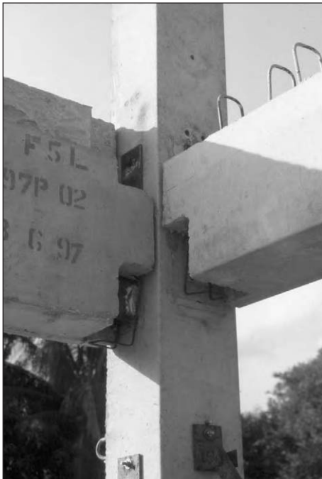
Figure 9.1: Beam-to-column face connections. Asymmetrically loaded beams require couple connections to prevent beam twisting.
