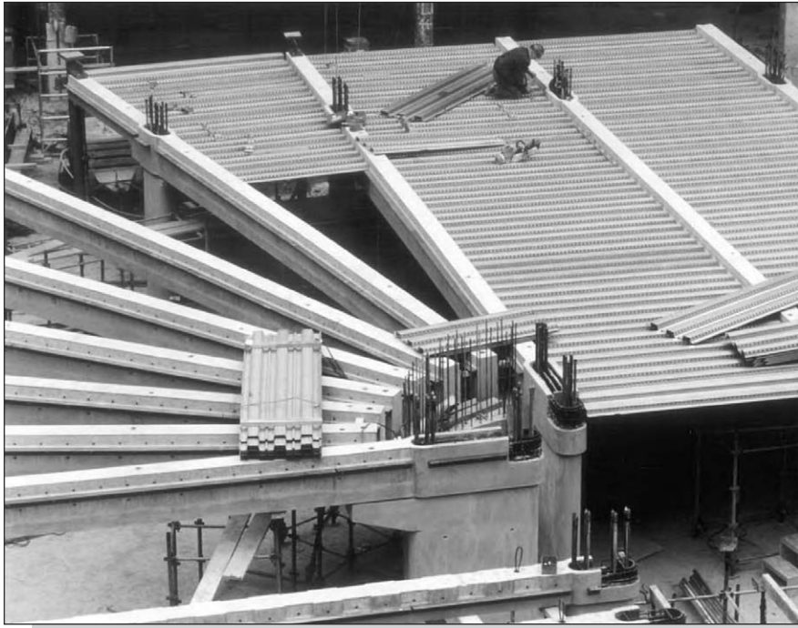
Figure 1.12: Mixed cast in situ and precast concrete, with composite steel decking floors (courtesy Trent Concrete, UK).
