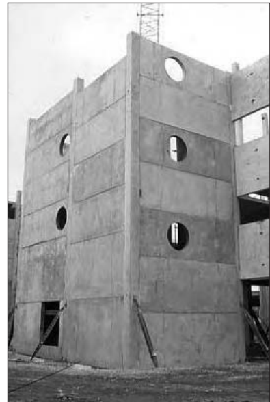
Figure 6.19: Precast concrete infill walls.
