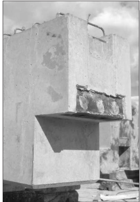
Figure 9.16: Recessed beam end connection to rectangular beam.
