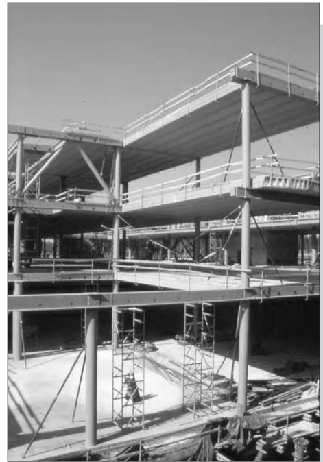
Figure 1.11: Mixed precast and structural steelwork construction.
