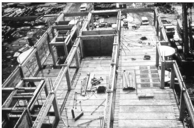
Figure 7.1: Precast concrete hollow core floor diaphragm in multi-storey construction (courtesy Reinforced Concrete Council, UK).
