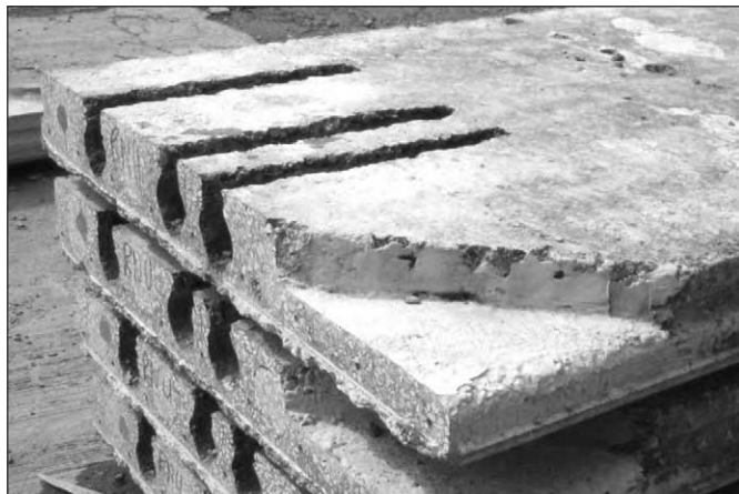
Figure 10.6: Corner recess in hollow core slabs to permit the correct placement of ties at corners.
