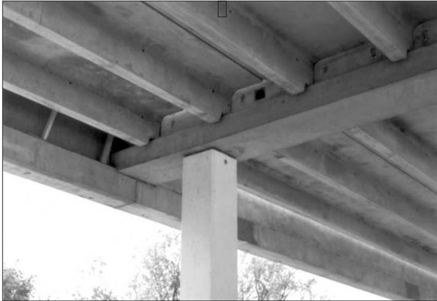
Figure 9.2: Beam-to-column head connections. A bearing pad and grouted dowels are also present.
