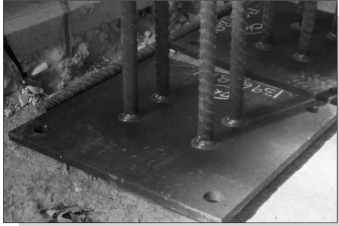
Figure 9.47: Starter bars welded to extended base plate.
