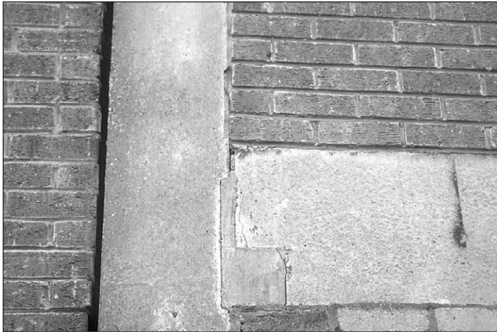
Figure 9.24: Shrinkage and other movement cracks around the edges of grouted up recesses.
