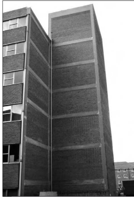
Figure 6.21: Brick infill shear wall.
