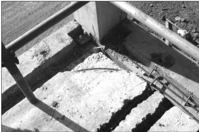
Figure 10.5: Continuity of beam ties at corner columns.
