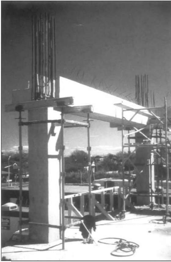
Figure 8.31: Moment continuity reinforcement placed in precast U-beams.
