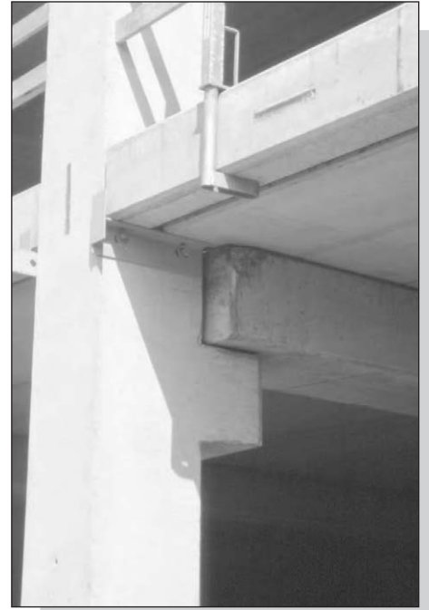
Figure 1.3: Simple bearing nib.
