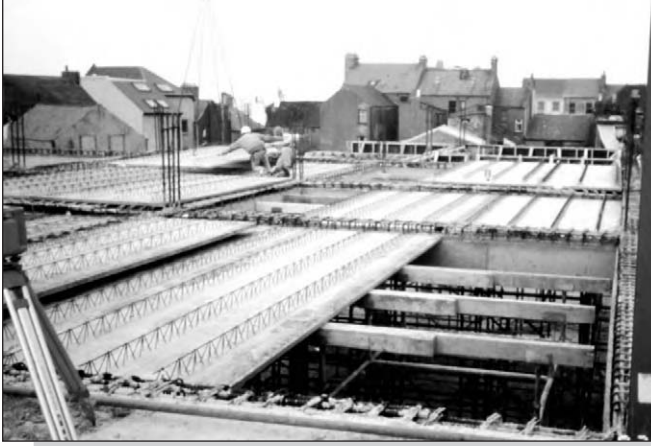
Figure 4.26: Propping of composite plank floor.
