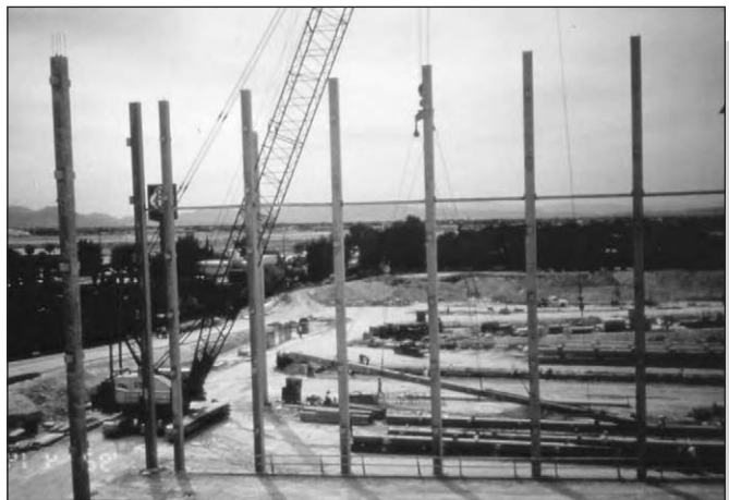
Figure 6.3: 25 m long single piece columns at MGM car park, Las Vegas (courtesy Andrew T Curd & Partners, USA).
