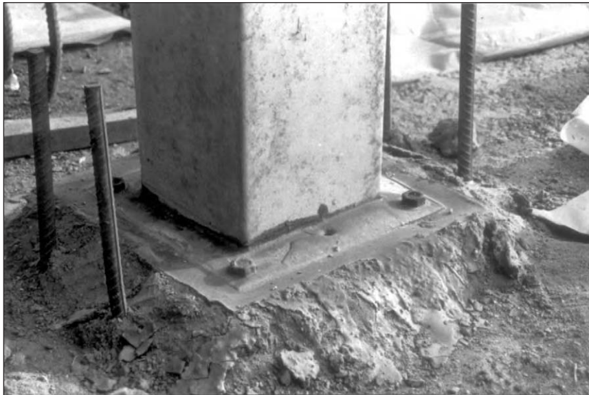
Figure 9.3: Column-to-foundation connection using extended steel base plate.
