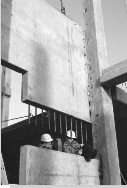
Figure 6.32: Horizontal interface shear reinforcement and vertical welded joints in an infill wall.
