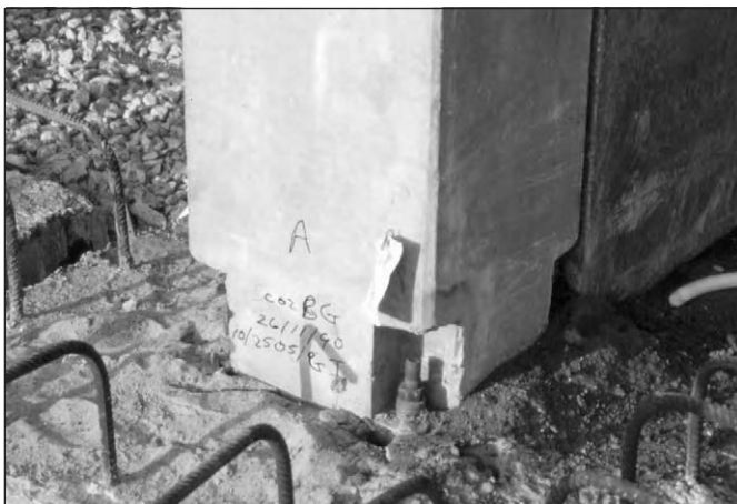
Figure 9.43: Column-to-foundation connection using flush steel base plate.
