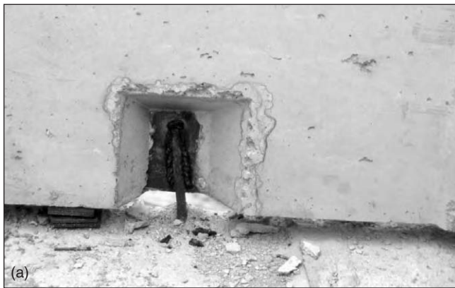
Figure 8.23a: Welded connection between rebar and plate.
