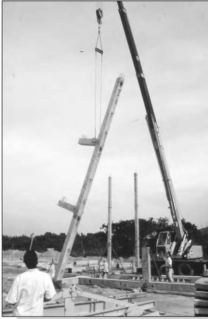
Figure 6.9: Pitching asymmetrical columns.
