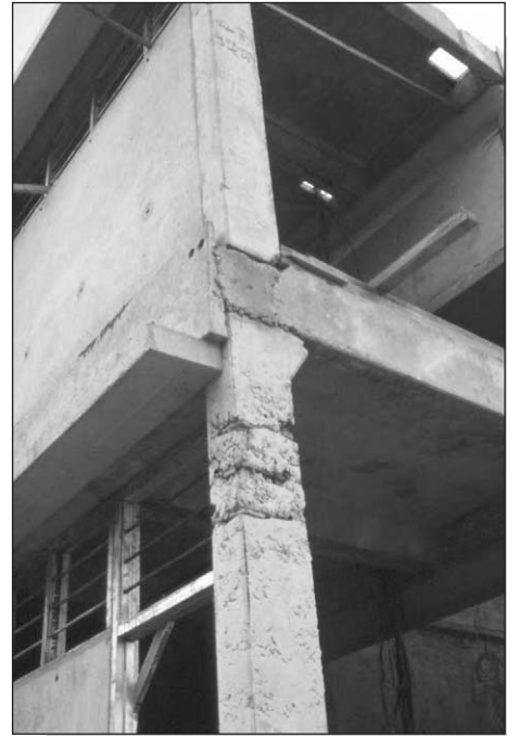
Figure 2.2: Compaction problems in a precast concrete column.
