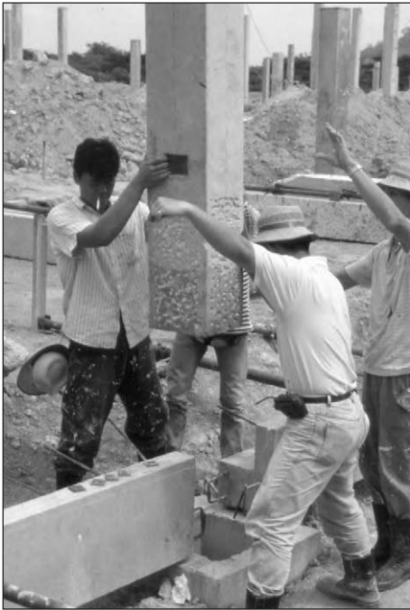
Figure 9.4: Column-to-foundation connection using grouted pocket.
