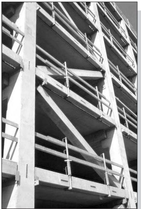
Figure 6.23: Concrete strut diagonal bracing.
